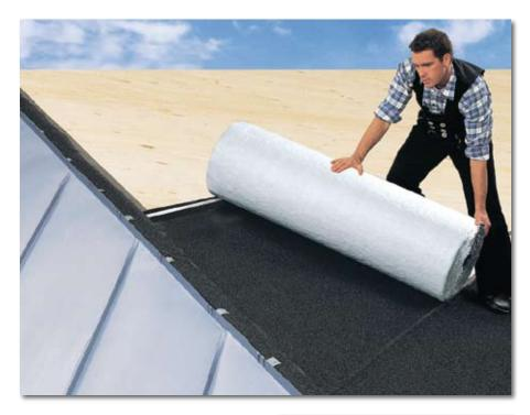
Permo® sec is a vapour permeable waterproofing barrier that is installed as a separating layer between copper, zinc, aluminium and stainless steel standing seam roof finishes and the supporting deck.
