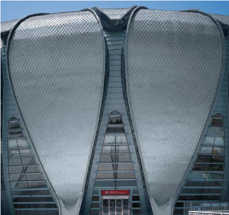
Olympic Stadium, Jinan, China
