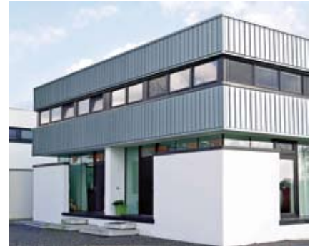
Building renovations, storey add-ons
